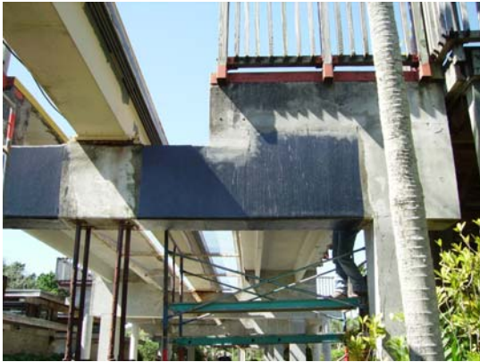
Application of Fiber Carbon Reinforced Polymer Straps
