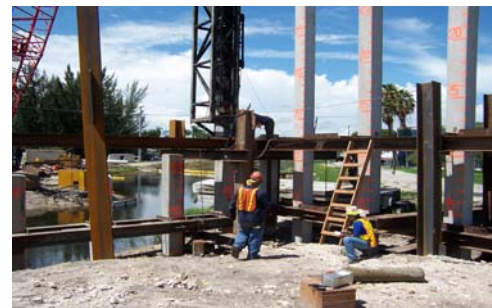
Pile Driving Operations for Bridge Foundation Contractor: Astaldi Construction Corp.
