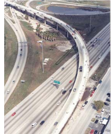
Work Progress Photo Contractor: Astaldi Construction Corp.
