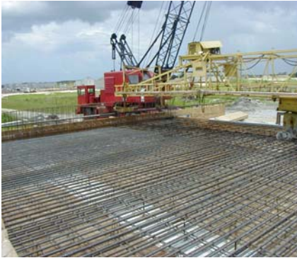
Reinforcing for Bridge Deck
